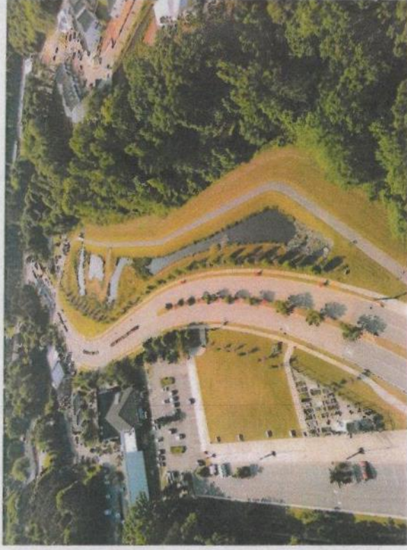
Example: Town of Morrisville Town Center - Stormwater Wetland (looking east) May 23, 2022
